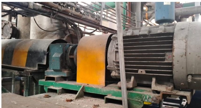
Figura 13 Componentes ROTOFORMER Motorreductor-Eje
