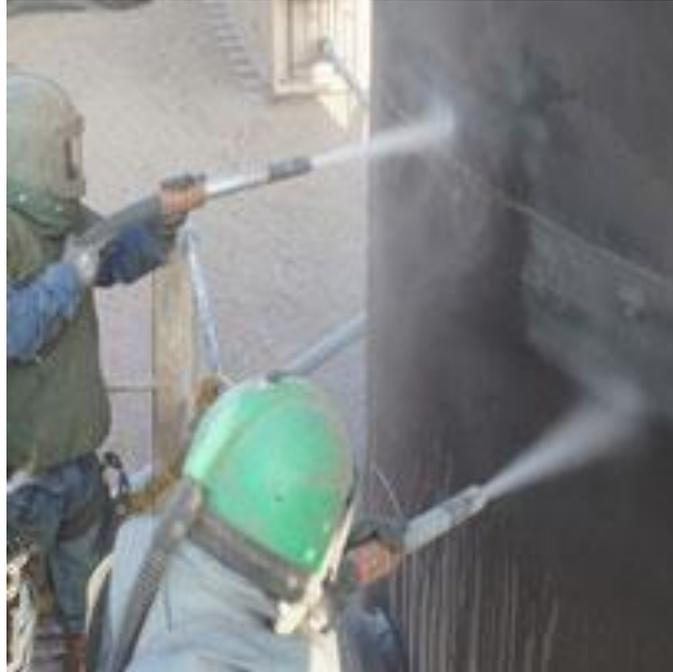
*Figura 7. SSPC-SP-7 / NACE N°4. Fuente: (CONSTRUCTORA OCITRIMEX, n.d.).*
